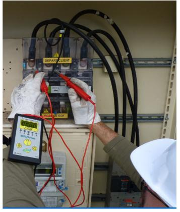
The instrument is **CAT IV**, (480V/2KAmps) and is weather/dust proof to **IP55**. It is built to -
